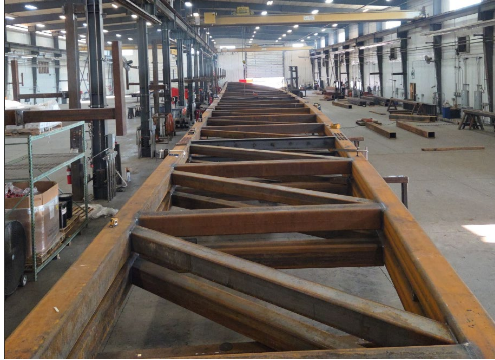
Photo 10. Fabrication of the new 265-foot-long clear span steel truss bridge in Loveland, Colorado.
