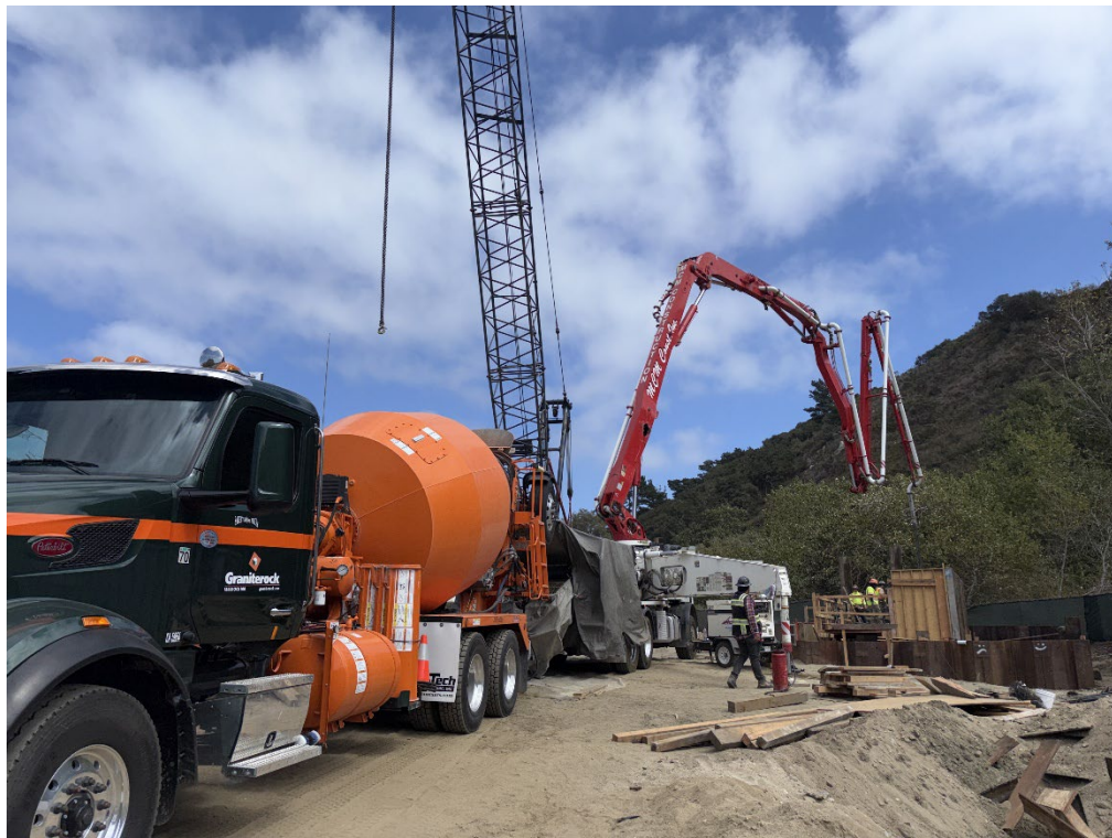
Photos 9. Concrete truck pouring the final concrete lift of the bridge abutment.
