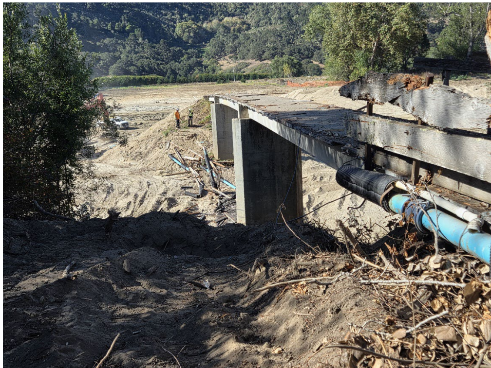
Photos 4 & 5: Demolition of Bridge #2 over the mainstem of the Carmel River.
