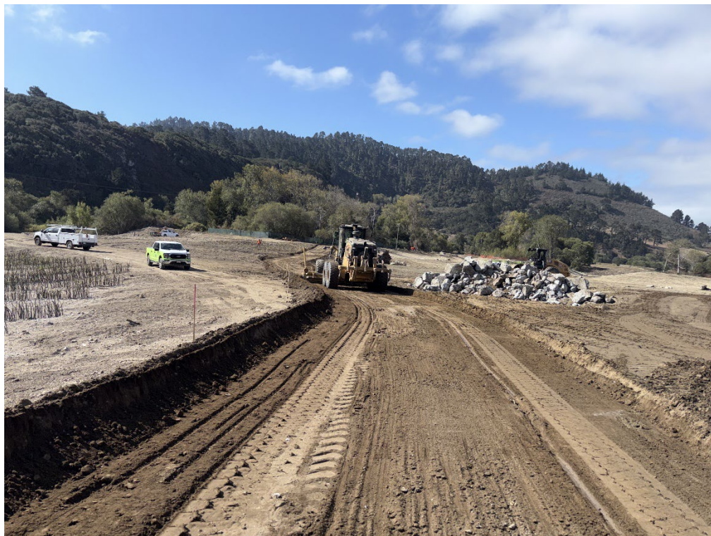
Photo 11: Rough grading of a new operations access road and public trail connection across the lowered floodplain.
