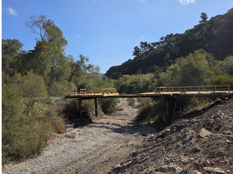
Photos 8. Looking upstream at a temporary structure to support installation of the new bridge.
