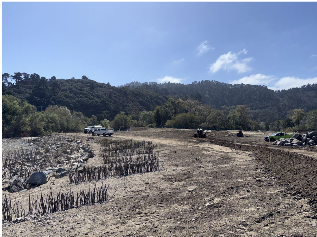
Photos 6 & 7: Installation of the IC channel widening, bank armoring, and willow pole cuttings.
