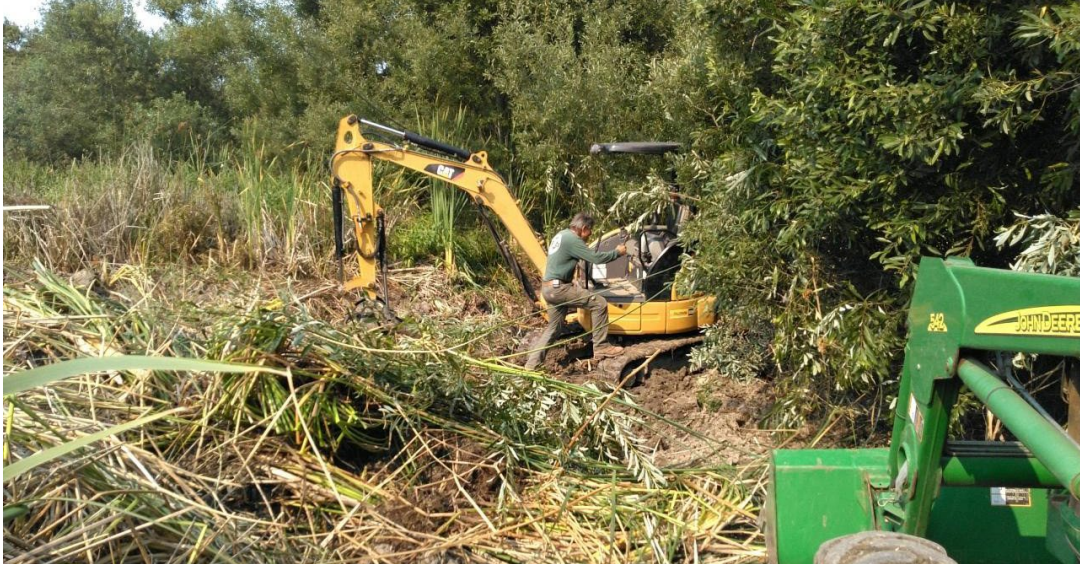
Ranger John removing tullies using the excavator
